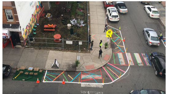
Painted curb extension and flexible delineators can be installed during the pilot project phase
