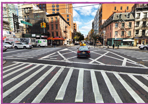
Box pavement markings at intersection
