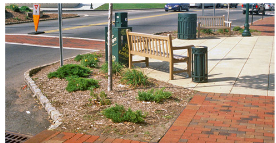
Curb extensions provide an opportunity to add pedestrian amenities such as benches and landscaping
