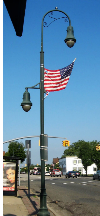
Pedestrian-scale lighting can be attached to same pole that provides light for traffic to save space
