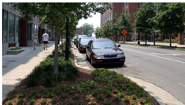
Curb extensions (aka Neckdowns) can be used to calm traffic in neighborhood slow zones. (Source: www.pedbikeimages.org/ Dan Burden)
