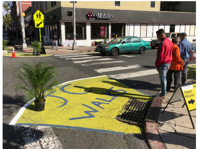
Painted curb extension and flexible delineators can be installed during the pilot project phase
