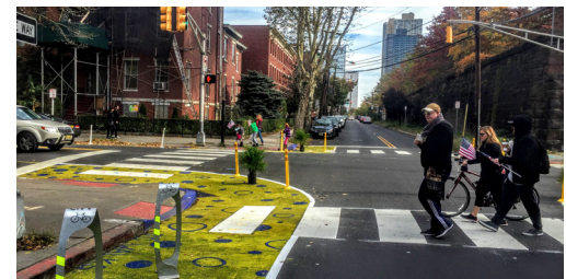
Painted curb extension and flexible delineators can be installed during the pilot project phase
