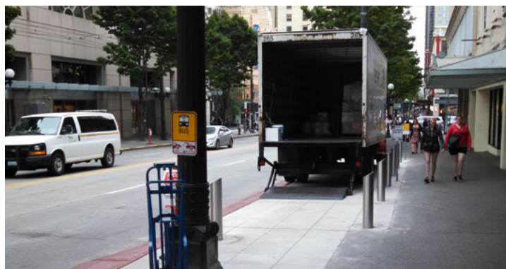
Dedicated space for truck loading zones can be incorporated into the sidewalk
