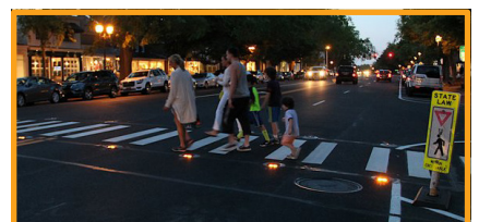
In-pavement crosswalk lighting
