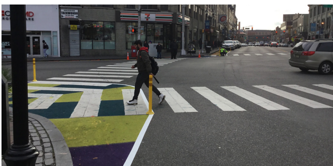
Painted curb extension and flexible delineators can be installed during the pilot project phase
