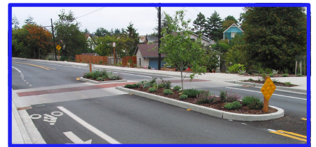
Raised crosswalk with pedestrian refuge
